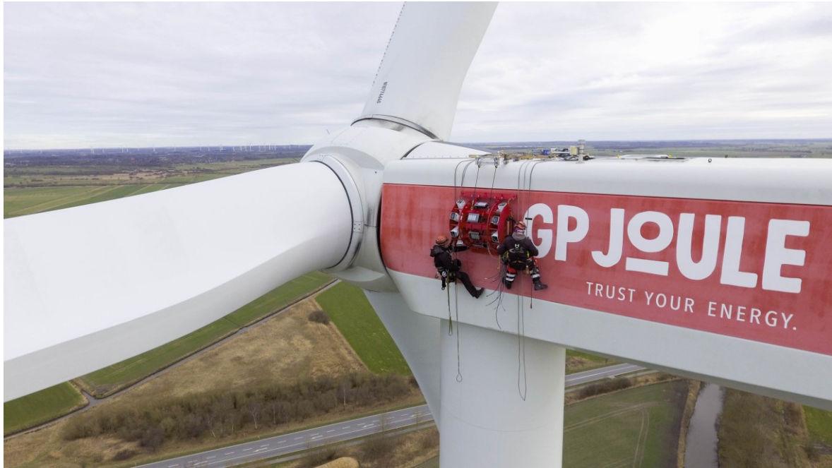
Figure 3-7 Installation of an AVES Offshore HPC system at the study site.
